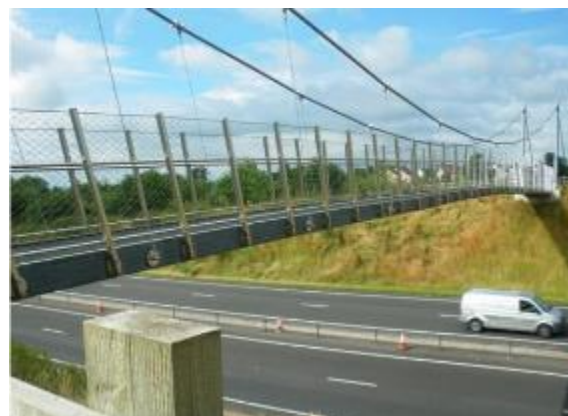
A5 Nesscliffe Bypass: New Footbridge over A5
