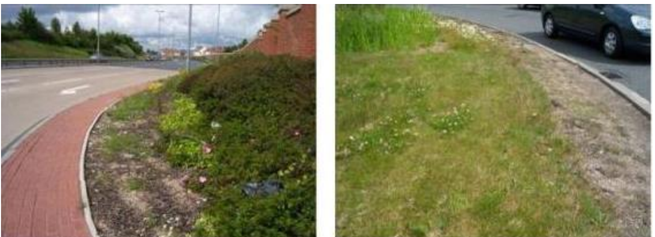
Figure 7-14 Examples where a splash strip was or was not provided at edge of kerb
