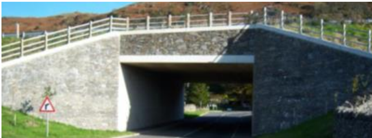
Figure 7-6 Stone faced headwalls at new culvert/mammal tunnel below the A590 High and Low Newton Bypass
