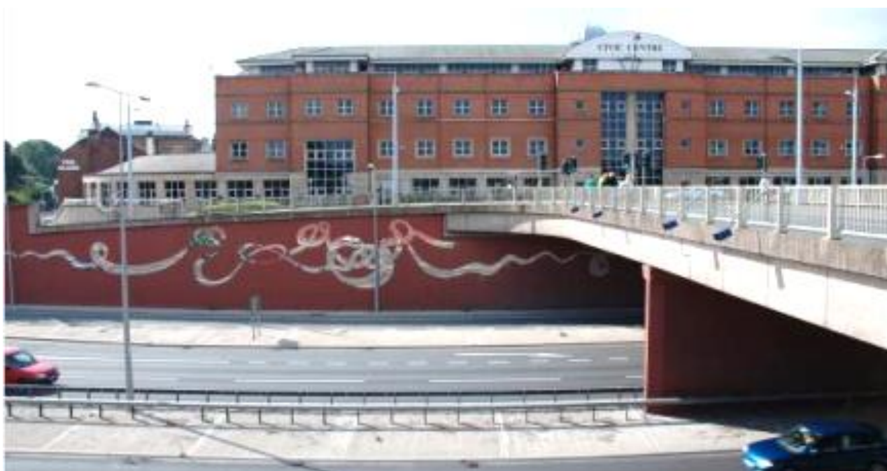
Figure 7-10 Concrete retaining wall cladding
