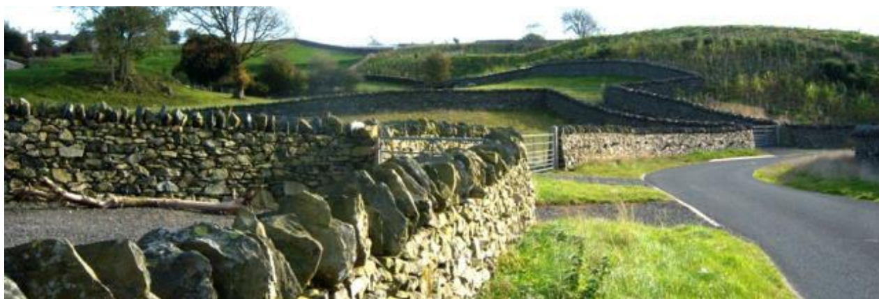
Figure 7-4 New dry stone walls replicate local boundary patterns, reuse field gateposts and tie into existing walls
